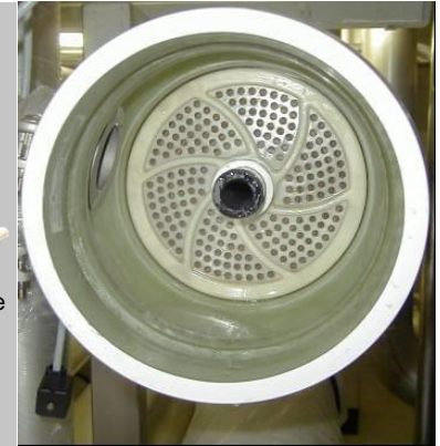
Detail of pressure vessel
